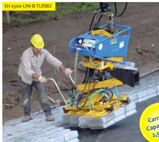
Illustration above: Installing deck stones with a special suction plate
