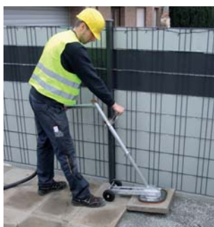
FXES-25 when laying concrete slabs outdoors
