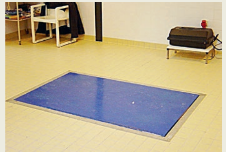
Lift table installed in a pit.
