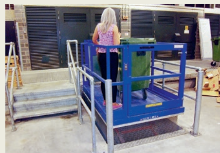
Lift table for goods and carriage of passengers.
