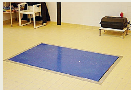
Lift table installed in a pit.
