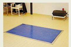
Lift table installed in a pit.
